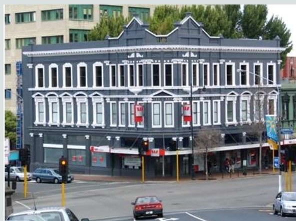
Crown Clothing Co building, cnr Frederick & George Sts, 2010.
